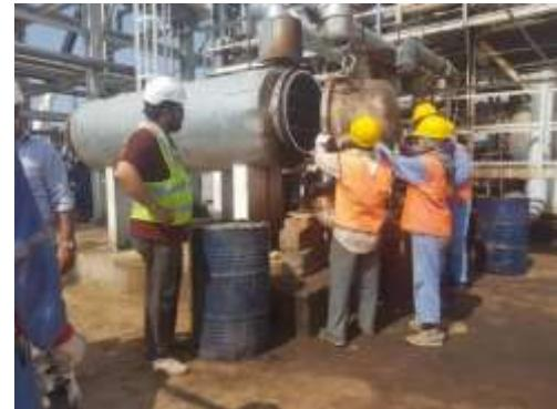
**Instrument:** Dismantling, shifting to workshop, refurbishment, inspection, lapping, calibration, pressure testing, parts replacement, re-tubing, shifting to plant area from workshop, re-installation & box up and commissioning of Control Valves ,PSVs and Transmitter at Chanda Plant
